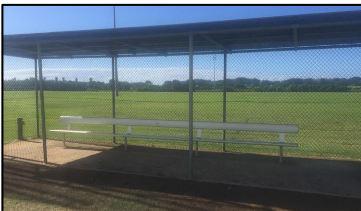
Field-level Dugouts – North Dalton Park, Wollongong
