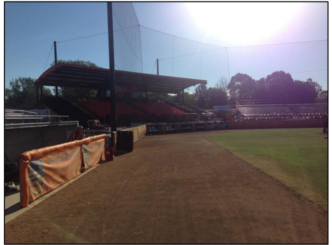
Net and cable backstop – Narrabundah Ballpark, Canberra
